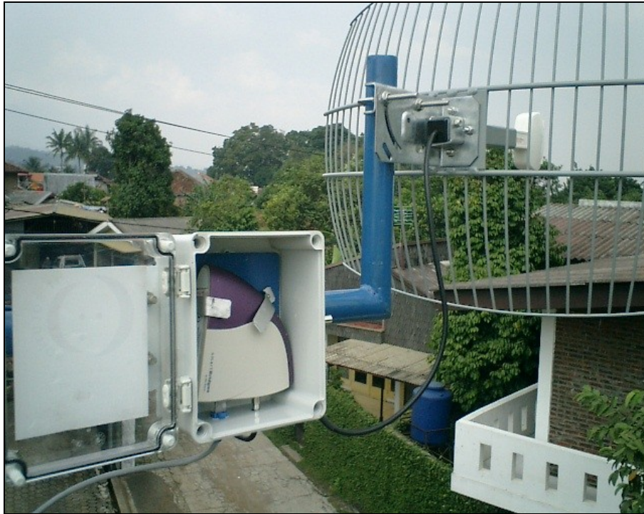
Image 21: Installation of a WiFi CPE
