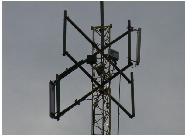
Image 17: Horizontal Isolation in a tower
