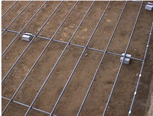
Image 6 a) Using Dobbies to create space between re-bars and the soil. b) Using wires to tie the re-bars to a grid. Source: http://www.do-it-yourself-tower.com/
