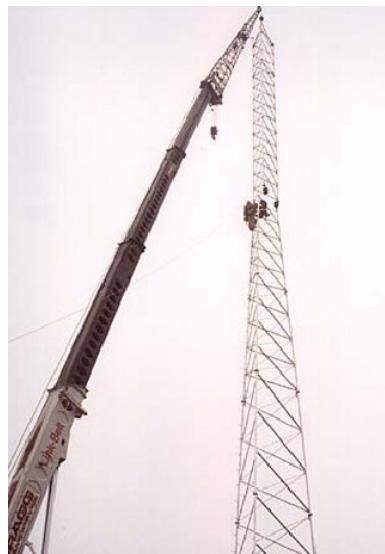
Image 9: Using a crane to place the top segment on a high self-supporting tower.
