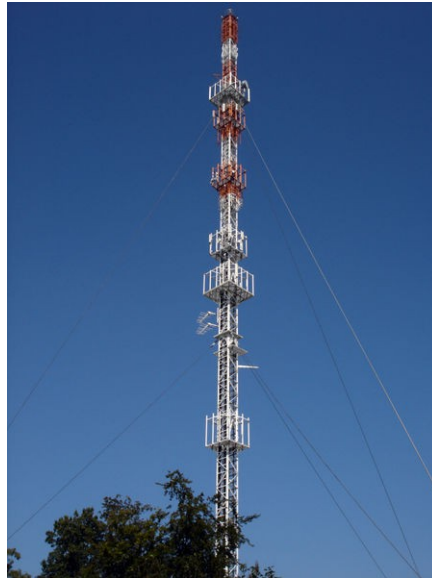
Image 14: A guyed mast with a total of six guy wires (two levels with 3 guys each).
