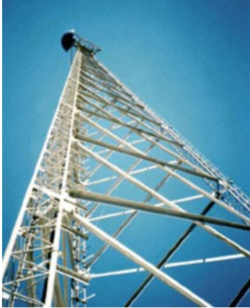
Image 3: A self supporting tower with no need of guys.
