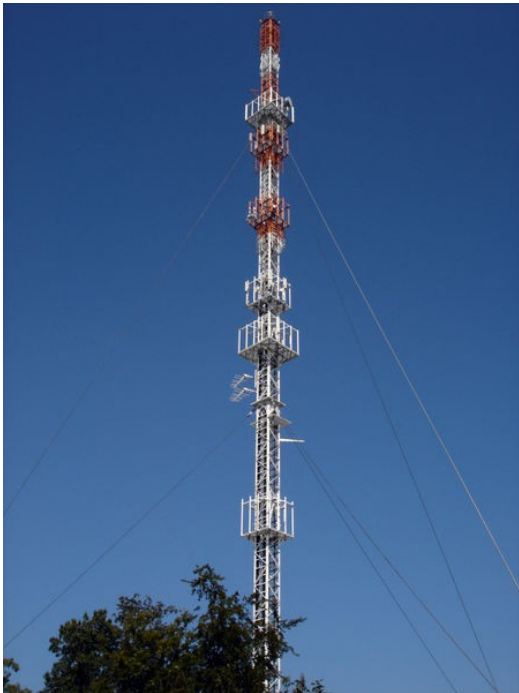
Image 4: A guyed mast with two level of guys attached in three points each.
