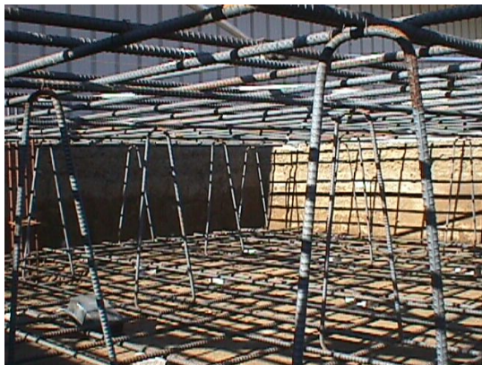
Image 7: a) Two layer of re-bars inter-connected with standees. b) J-Bolts that will connect the base of the tower to the concrete foundation.
