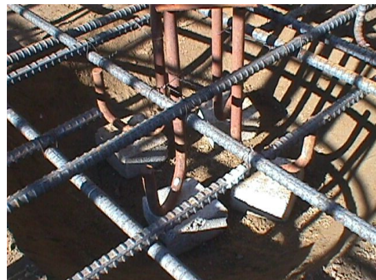
Image 7: a) Two layer of re-bars inter-connected with standees. b) J-Bolts that will connect the base of the tower to the concrete foundation.
