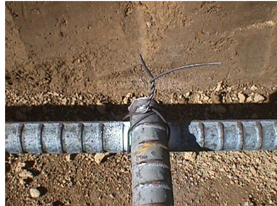
Image 6 a) Using Dobbies to create space between re-bars and the soil. b) Using wires to tie the re-bars to a grid. Source: http://www.do-it-yourself-tower.com/
