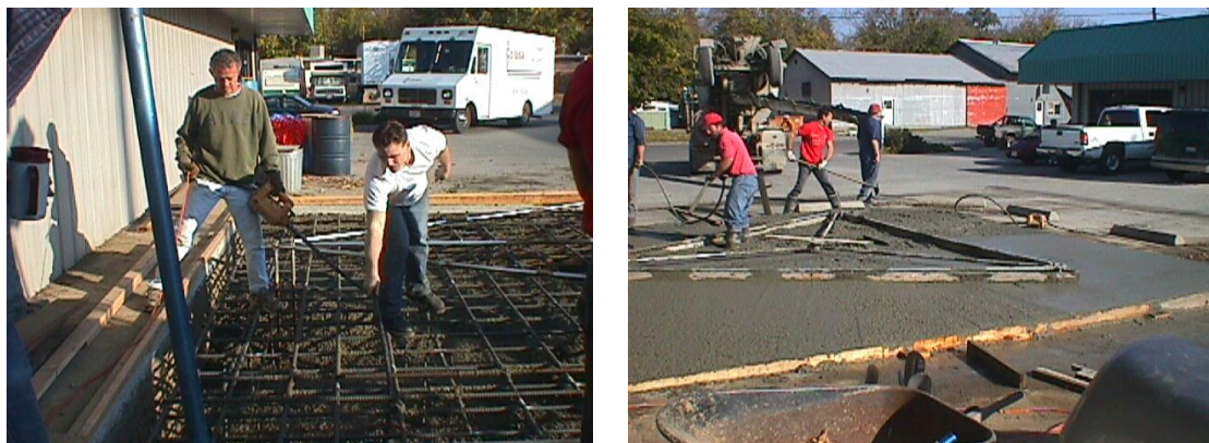
Image 8: a) Using a vibrator in the wet concrete to eliminate flaws such as honeycombs and air pockets. b) The central area should be flat with a brushed finish while the surrounding area is sloping (outwards) with a floating finish (completed only in the right corner).
